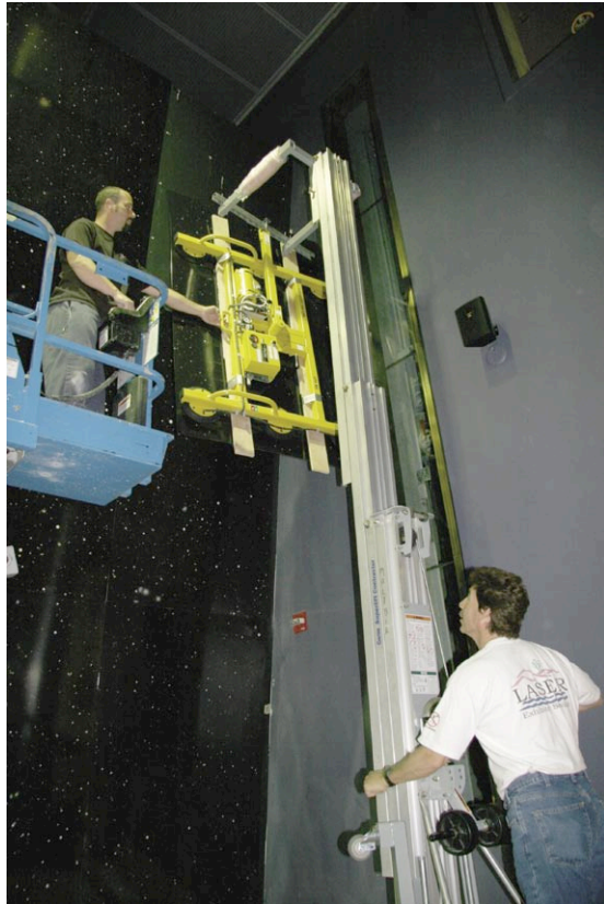
The upper panels were installed using a lift equipped with those suction cups you normally see in bank-heist movies when a plate-glass window needs to be cut.
